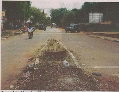
A road in Moroto. Photos by Olandason Wanyama
